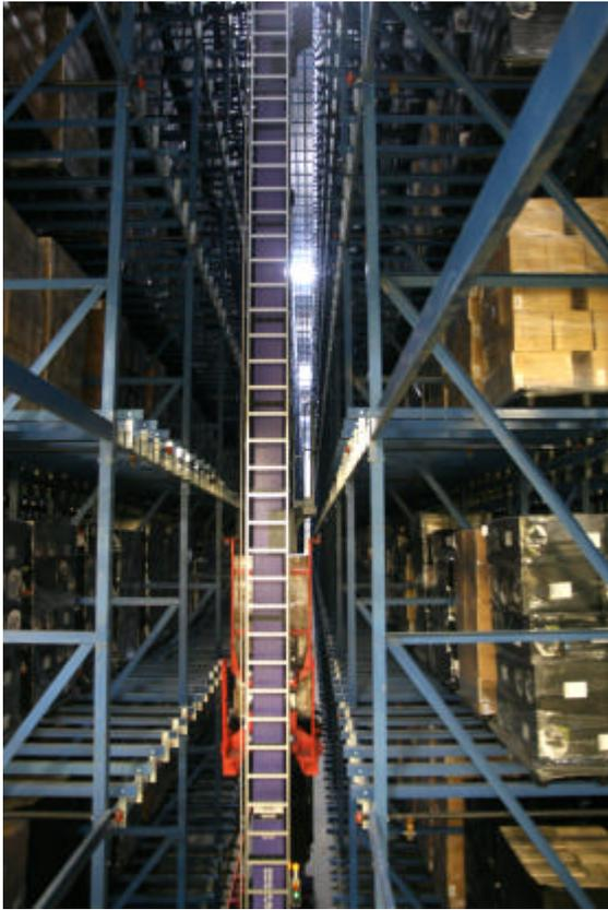
the rack is incorporated into the actual building and serves as its basic structure while seamlessly integrating with the material handling system.
