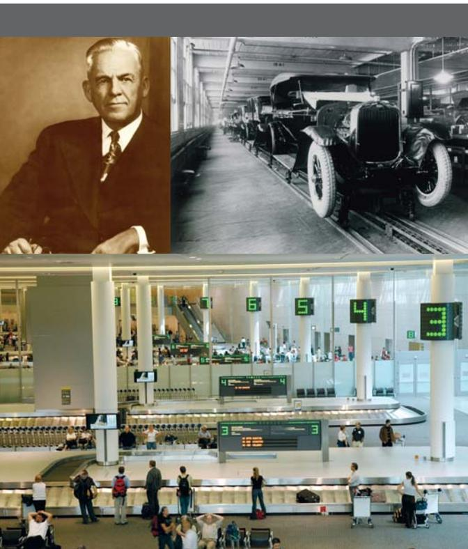
Since 1919, the Jervis B. Webb Company has been at the forefront of the material handling industry. Our founder Jervis B. Webb adapted a forged rivetless chain conveyor used in the mining industry to the rugged needs of the automotive industry, allowing automobiles to efficiently move on an assembly line. This single invention helped revolutionize mass production.
