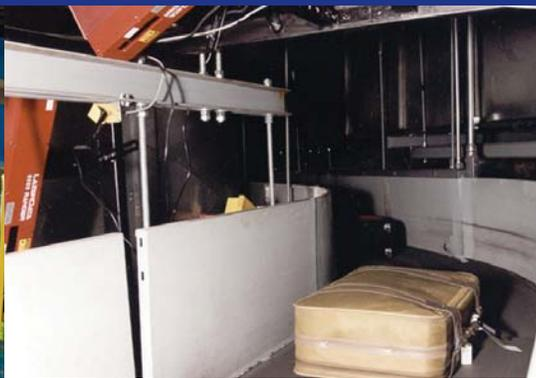
Laser scanners read bag tag barcodes to determine the destination flight and assigned make-up location in order to activate in-line bag sorters.
