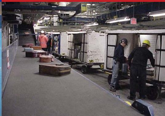
Inbound baggage is placed on belt conveyors that lead to the appropriate baggage carousels.
