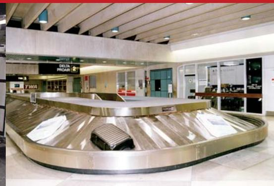
Arrival passengers can pick up their baggage from a quiet, heavy-duty sloped plate carousel (or a flat plate carousel).
