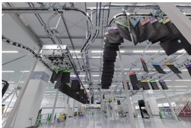
Rails installed in overhead space
