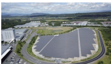
52,000 square meters of solar panels
