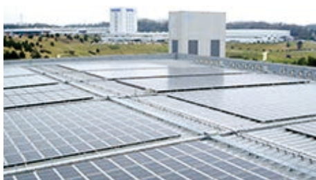
Solar modules installed on the rooftop
