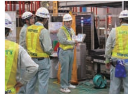
Top management conducting a safety patrol at an installation site
