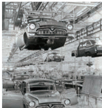
Chain conveyor system delivered to Japan's first passenger automobile factory (Page 5)
