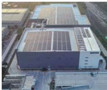
Photovoltaic system installed on the roof of manufacturing facilities for our cleanroom systems (Suzhou, China)
