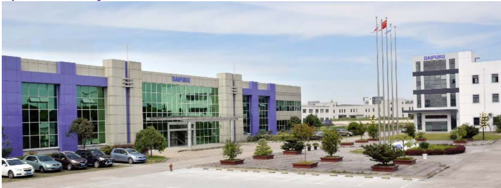
New head office and factories of Daifuku (China) Manufacturing Co., Ltd.
