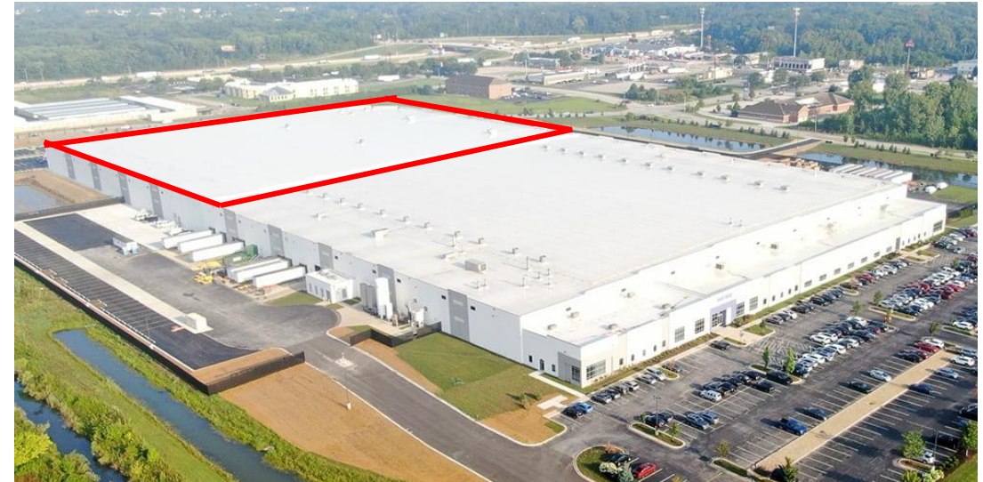
The expanded Hobart manufacturing plant
