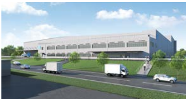
New facility within Shiga Works (rendering)
