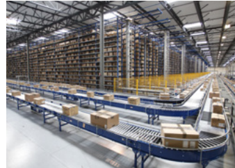
Integrated Conveyors and AS/RS
