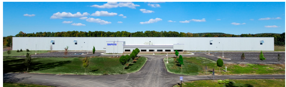
Northern Michigan Manufacturing Facility
