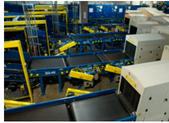
Baggage Handling Systems
