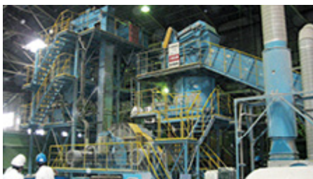
Site review conducted by Daifuku employees
