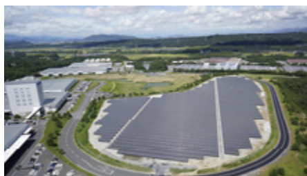
52,000 square meters of solar panels
