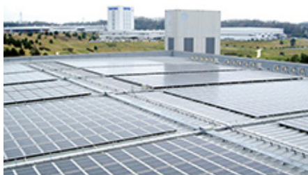
Solar modules installed on the rooftop
