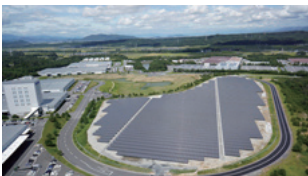
52,000 square meters of solar panels
