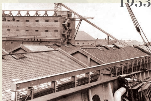
The first Bulkveyor installed
