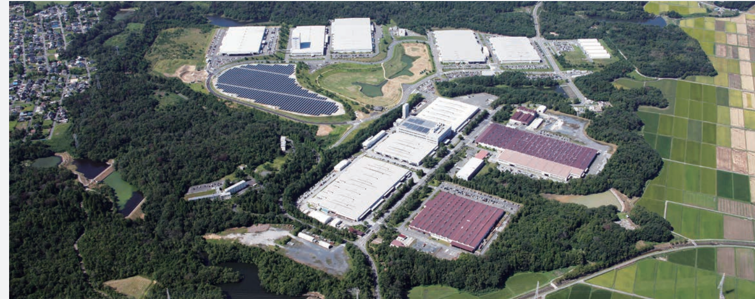
Shiga Works today
