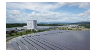
Daifuku Shiga Mega Solar 17,752 solar panels are installed on grounds measuring about 52,000 square meters. With a generating capacity of 4,400 kW, it produces 4.3 million kWh annually.
