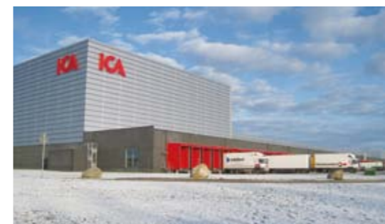
ICA's Helsingborg Distribution Center
