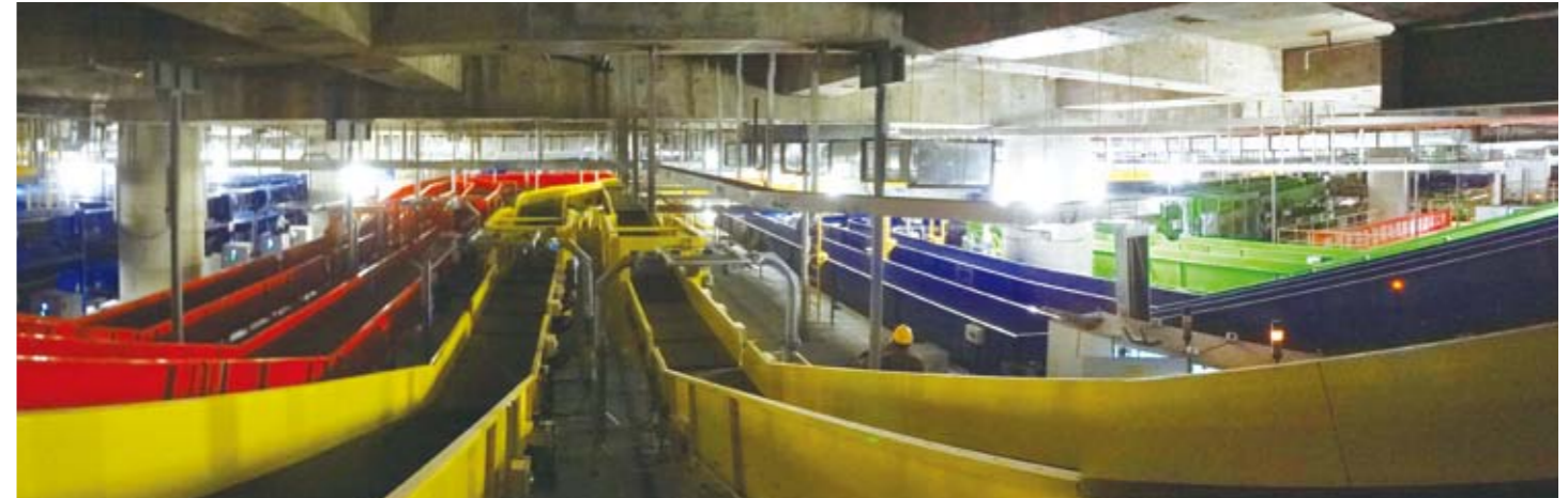
Sixteen check-in lines divided into four groups that are color-coded for easy recognition
