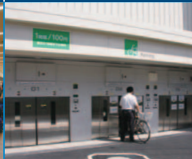
...bicycle parking tower operations near train stations
