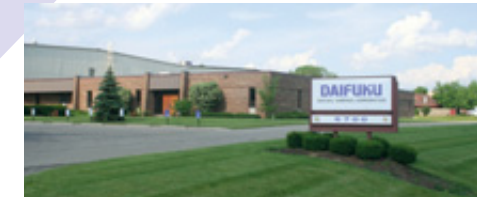
Daifuku America Corporation Ohio Plant
