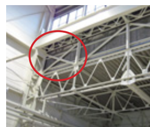
Additional reinforcement braces (Factory C, Shiga Works)
