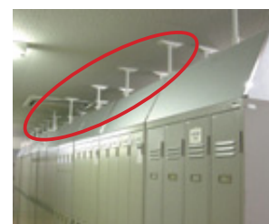
Office lockers anchored to prevent them from toppling over
