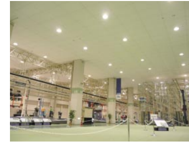
Mercury lamps were replaced with more efficient lamps on the showroom floor
