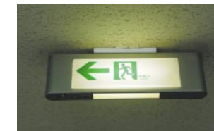
Emergency signs and lighting were replaced with LEDs
