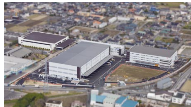
The Komaki Works houses five buildings within an approximately 56,000 square meter site
