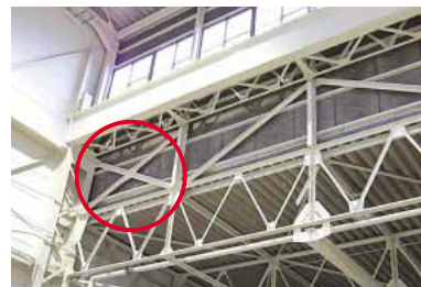
Reinforcement braces (Factory C at the Shiga Works)
