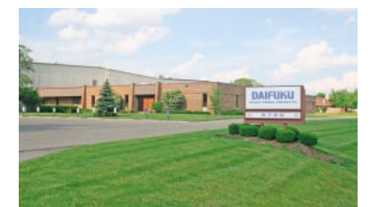
Daifuku America Corporation Ohio Plant
