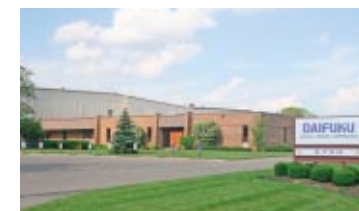
Daifuku America Corporation Ohio Plant
