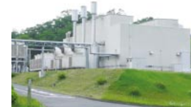
The Shiga Works cogeneration facility has been in operation since 1997
