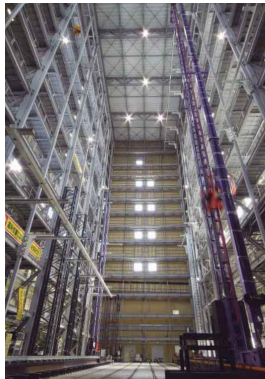
Interior view of R&D tower, Shiga Works
