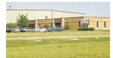
● Daifuku America Corporation Ohio Plant
