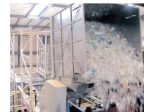
The recyclable waste retrieved from unit load AS/RS is introduced to a volumetric feeder unit utilizing a reverse function
