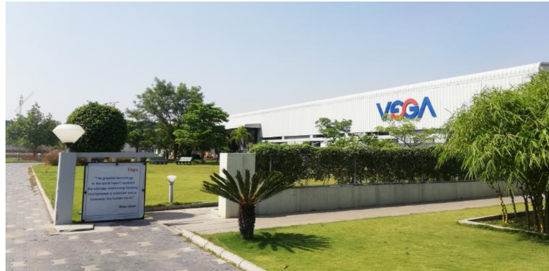
Vega Conveyors and Automation's main office and factory (Hyderabad, India)
