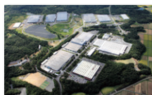
Shiga Works (Main Campus)
