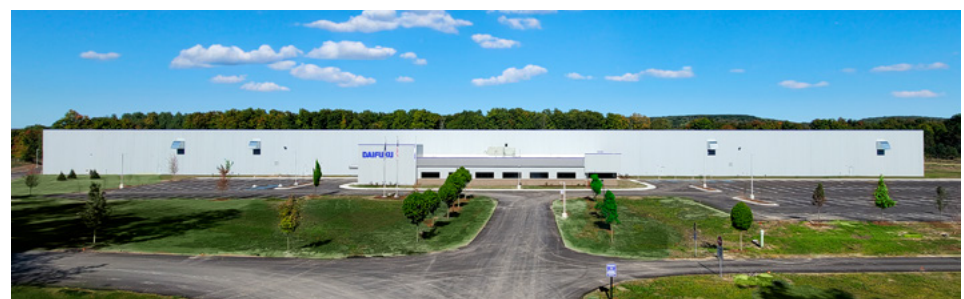
Northern Michigan Manufacturing Facility
