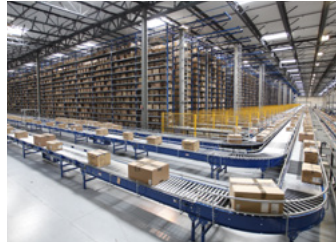
Integrated Conveyors and AS/RS
