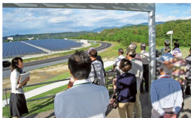
Shiga Works site tour for shareholders, viewing Daifuku's mega-solar facility
