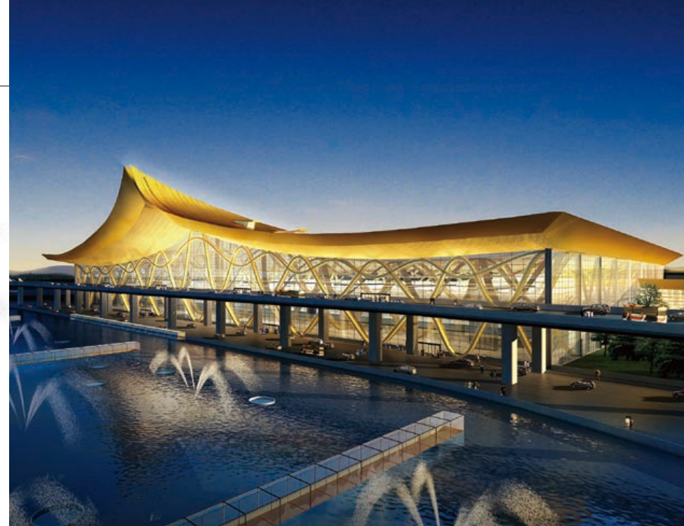
Daifuku Logan's baggage handling systems are used at Kunming Airport.
