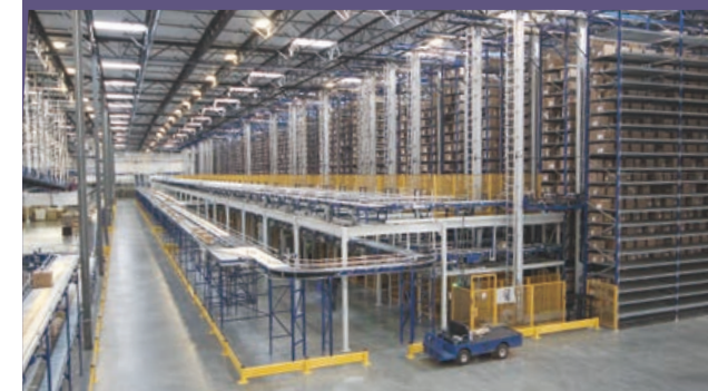
SKECHERS distribution center
