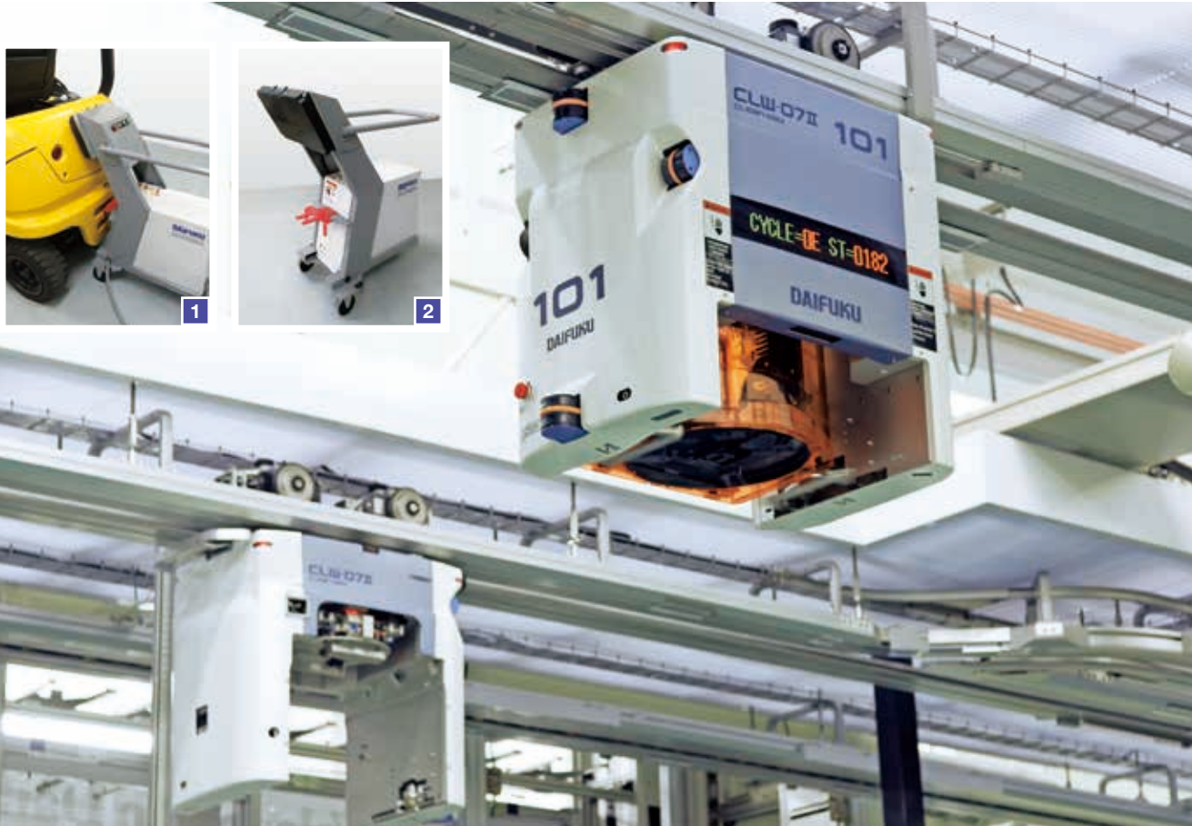
Overhead monorail system Cleanway using HID for semiconductor factories
