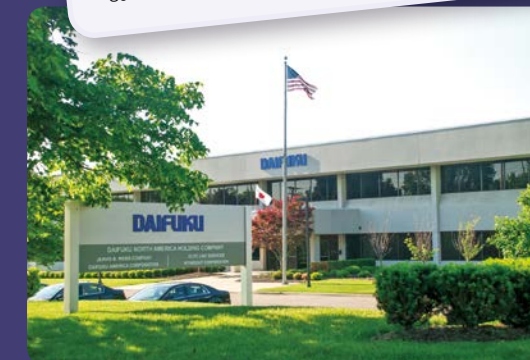
Daifuku North America Holding Company
