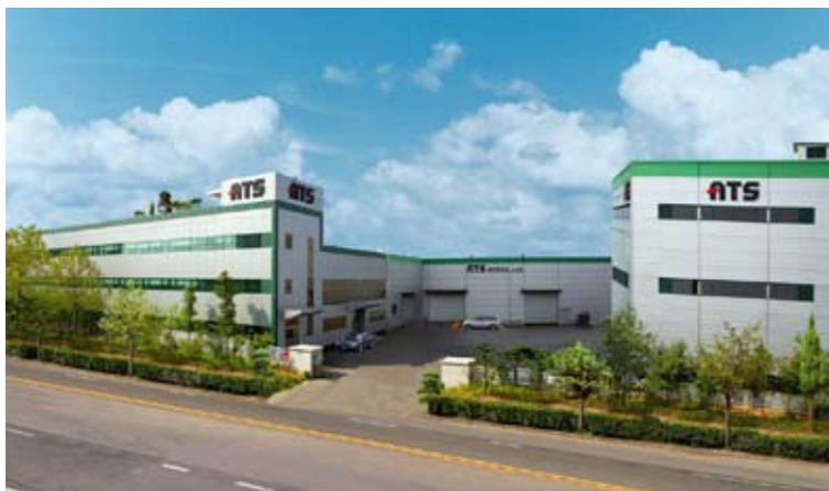
ATS head office and No. 1 plant
