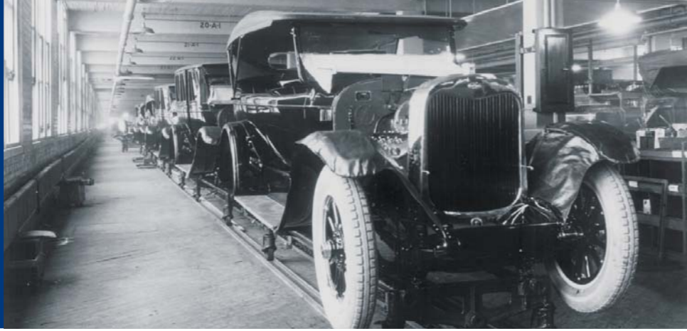
Webb's chain conveyor systems installed at Ford Motor Company in the early 20th century
