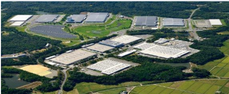
Panoramic view of current Works
